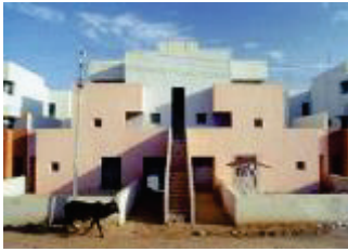
17 Residence in its original configuration before residents moved in: »Housing for Life Insurance Corporation« (LIC), Ahmedabad, 1973 © Vastushilpa Foundation, Ahmedabad
