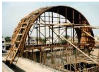
02 Construction of barrel-vault for Doshi's architectural studio, using traditional methods: »Sangath Architect's Studio«, Ahmedabad, 1980 © Vastushilpa Foundation, Ahmedabad
