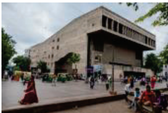
23 Exterior view of the concert hall: »Premabhai Hall«, Ahmedabad, 1976 © Courtesy of Vastushilpa Foundation, Ahmedabad, photo: Vinay Panjwani – India
