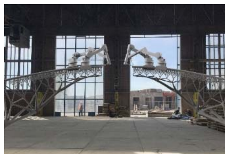
04 Joris Laarman for MX3D »Bridge Project«, 2015, 3D-printed pedestrian bridge © Joris Laarman Lab
